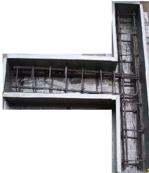
Fig. 6 Reinforcement details of beam-column joint
